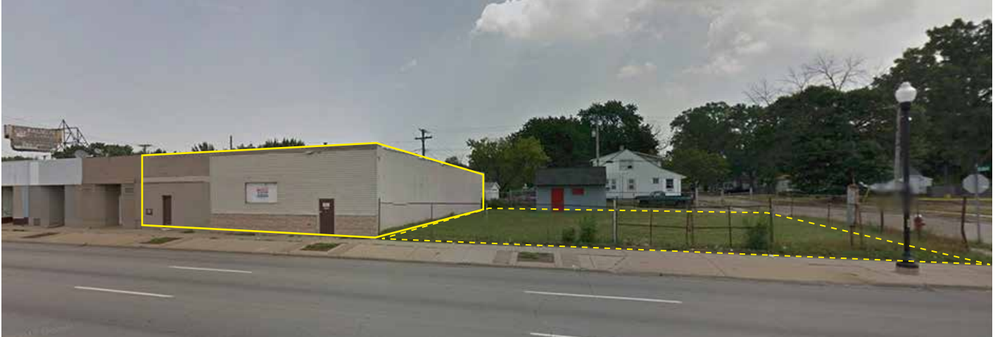
BUILDING EXTERIOR (VAN DYKE FRONTAGE) W/ADJACENT SIDE-LOT
