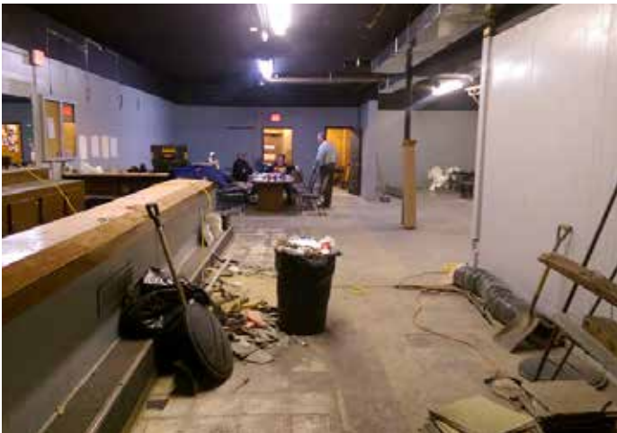
BUILDING INTERIOR (LEFT 1/3 FROM REAR (MAIN) ENTRANCE - ZONE 1)
