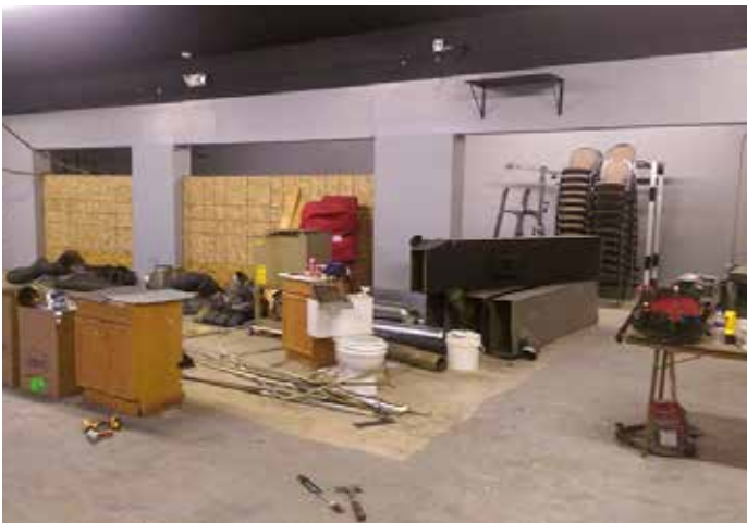
BUILDING INTERIOR (CENTER 1/3 FROM REAR KITCHEN SPACE - ZONE 2)
